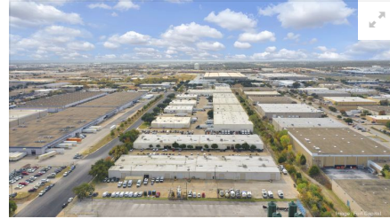
The Arden Group has acquired a 12-building, 582,803-square-foot industrial portfolio in North Texas.
